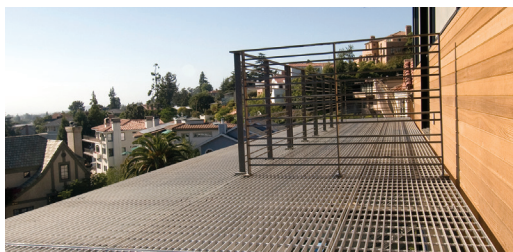
McNICHOLS® Bar Grating, Swage-Locked, GAL-100 - Sunshade, Margarido House, Oakland, CA
