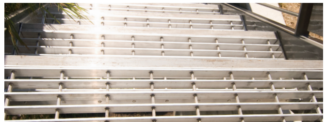
McNICHOLS® Bar Grating, Swage-Locked, GAL-150 - Stair Treads - Margarido House, Oakland, CA
