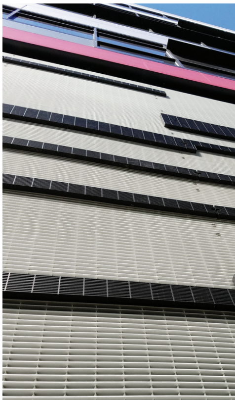
McNICHOLS® Bar Grating, Swage-Locked, GAL-150, and Press-Locked, GCM-1-150 - CLOSE MESH - Grocery Store Facade
