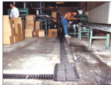
This distillery floor has been retrofitted with a presloped trench drain.
