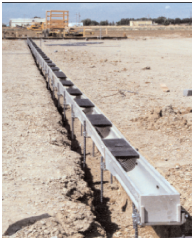
Photo shows the installation process of the durable presloped trench drain system.
