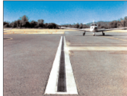
Optional heavy duty frame provides adequate drainage for this airport runway.
