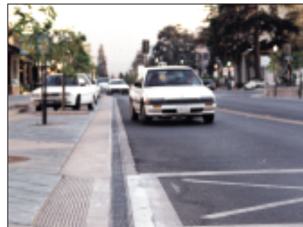
Trench drain handles the high flowrate needed for this municipality street area.
